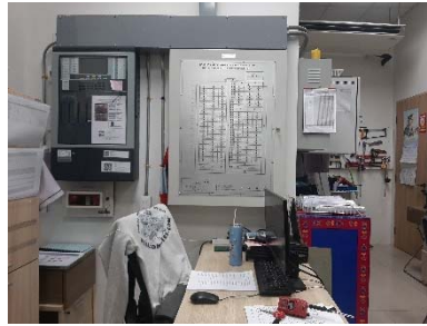
Graphic Annunciator Fire Alarm System
